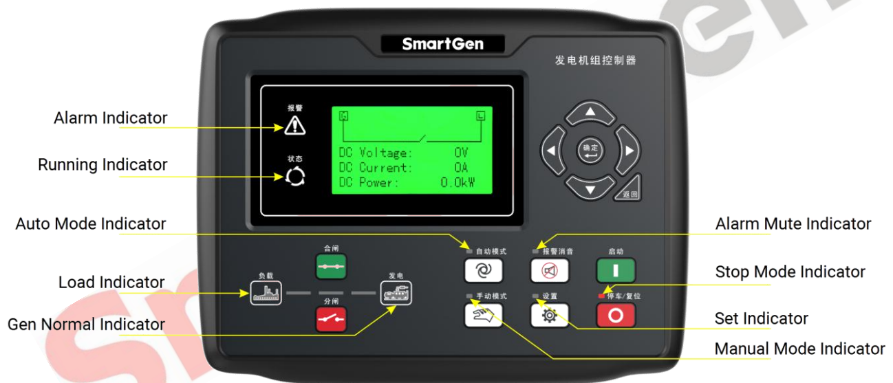
Fig. 1 - Controller Front Panel
